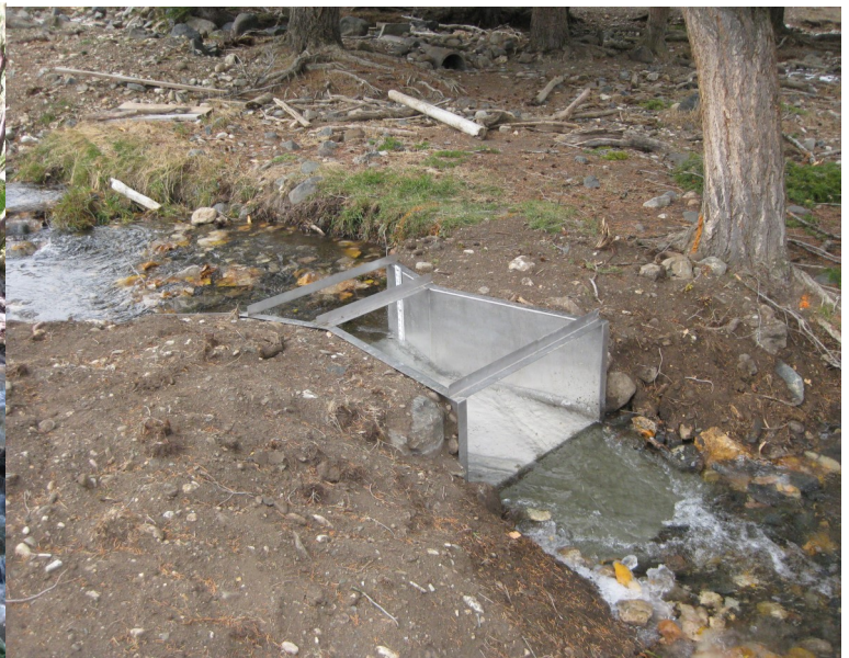
Flume installed to measure stream flow on the lower Rock Creek diversion
