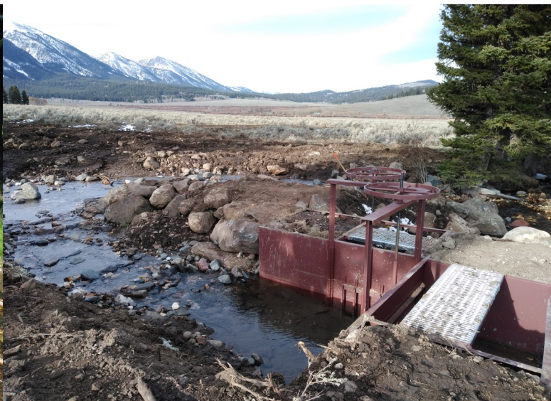
Lower Rock Creek after completion
