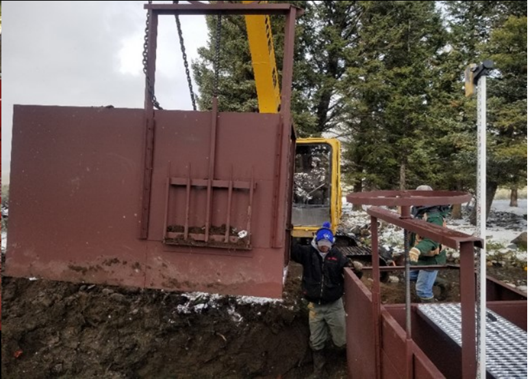
Rock Creek Lower Diversion Under Construction Darin Schneider IDFG Recreation Site Maintenance Foreman on Backhoe Louis Wasniewski, USFS Hydrologist in Green Jacket
