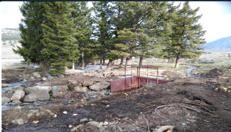
Rock Cr Lower Diversion after controlled head gate installation
