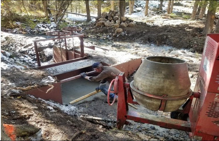
Lee Mabey, USFS completing cement on Upper Rock Creek
