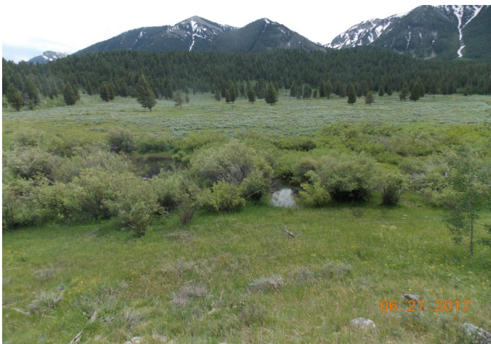
Close up pic of BDA structure . Summer 2017
