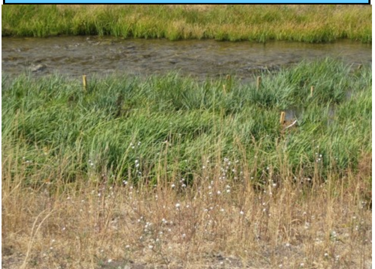
Sedge mats installed on Howard Creek
