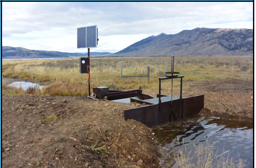
Built-in head gate integral to the design along with a traditional paddle wheel
