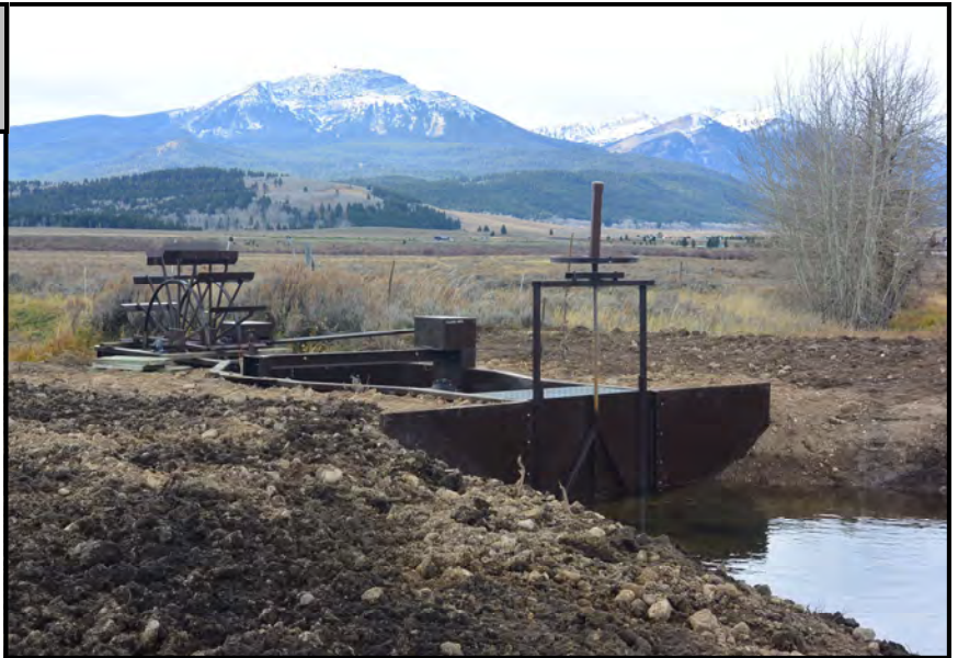
Built-in head gate integral to the design along with a traditional paddle wheel
