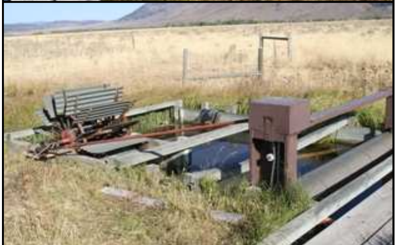
The last two old wooden diversion screens on Howard Creek at the pond just above the fish ladder that will be replaced this fall with the new modular steel screens.
