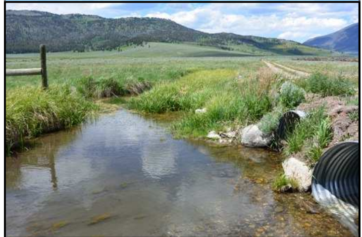
Poorly functioning culverts on Kelly Spring Creek
