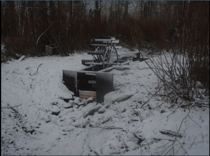
The new diversion screen installed. It got really cold and snowed hard by the end of the day.
