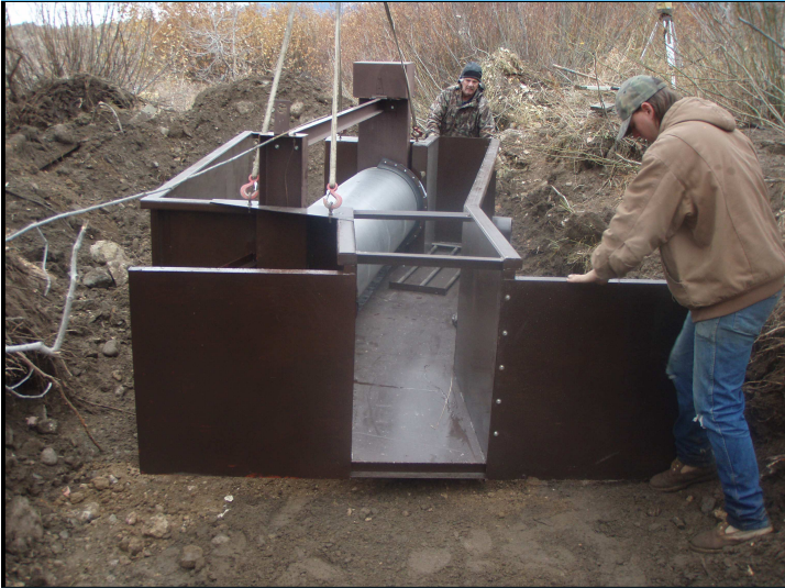
The new metal modular screen being lowered with IDFG Jim Parks (background of photo) directing the efforts.
