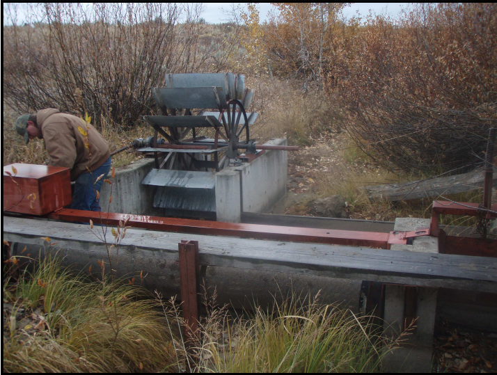
Old concrete and wood non-functioning diversion screen on the Cole property on Targhee Creek.
