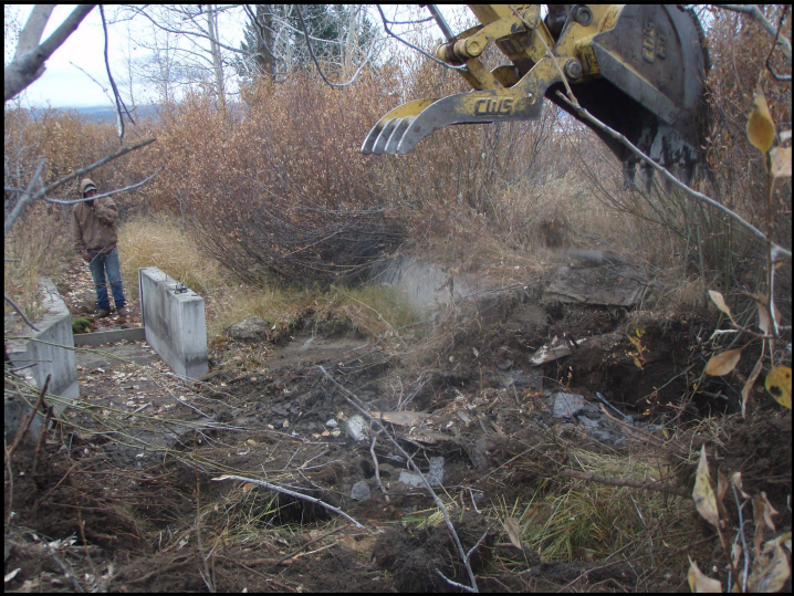
Larry Voss Construction removing the old structure from the site. The weather started out much better that day than it ended.
