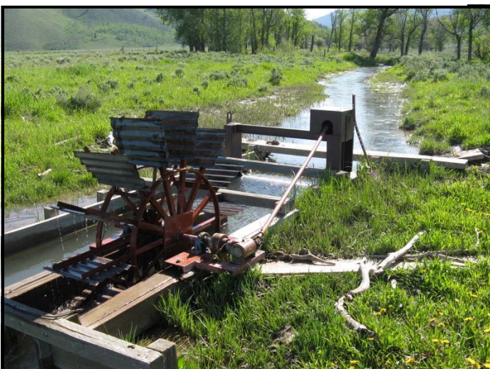
The old wooden diversion screen on the Salisbury property on Targhee Creek.
