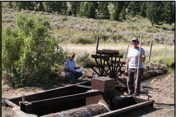
IDFG Fisheries Biologist Jessica Buelow and IDFG screen shop construction foreman Jim Hardy with the new modular steel screen.
