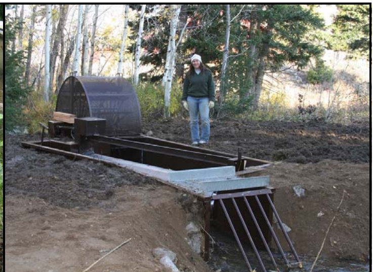
IDFG Fisheries Biologist Jessica Buelow with the new modular steel diversion screen on the Stockon property on Targhee Creek. This large 10' screen is now angled to the stream flow. The paddle wheel was also caged because of safety concerns.
