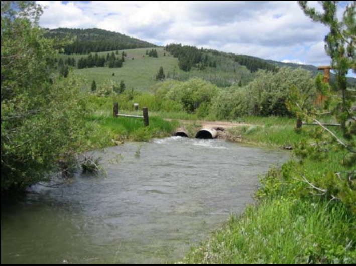
Double barrel culvert restricting cutthroat access at high flows
