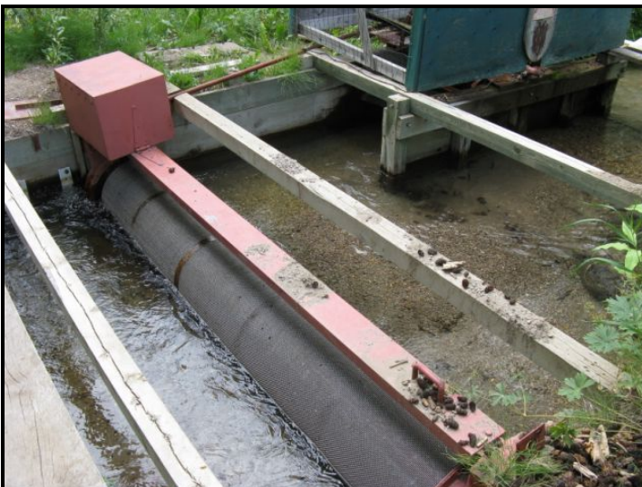
Old wooden diversion screen on the Stockon property on Targhee Creek. It was perpendicular to the stream and leaking underneath. Over 150 fry were found behind the screen and in the diversion ditch when it was removed. They were netted and released in Targhee Creek.
