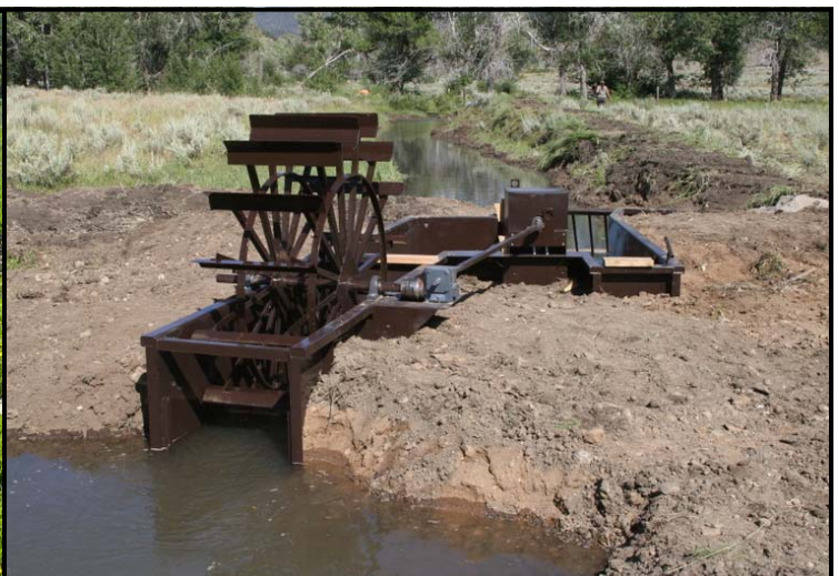
The new modular steel screen now installed in the same location.
