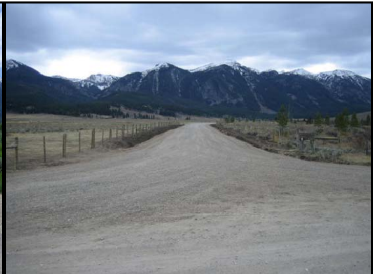
Post project with new section of Red Rock Road
