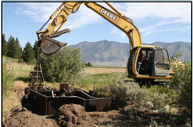
Installation on August 23 of new modular diversion screen on Parkinson property on Duck Creek.
