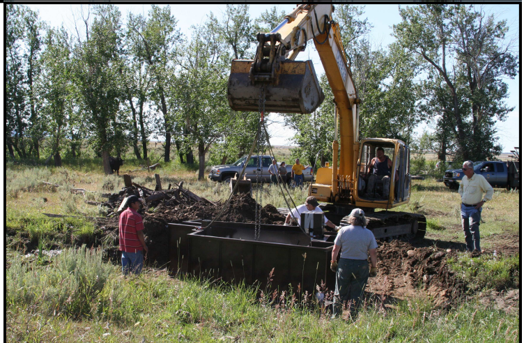
Installation on August 22 of new modular diversion screen on Salisbury property on Targhee Creek.
