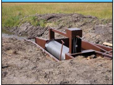
Above: New modular drum screen installed on Duck Creek on the Taft property. Below: One of the culverts on Duck Creek to be replaced later this year.
