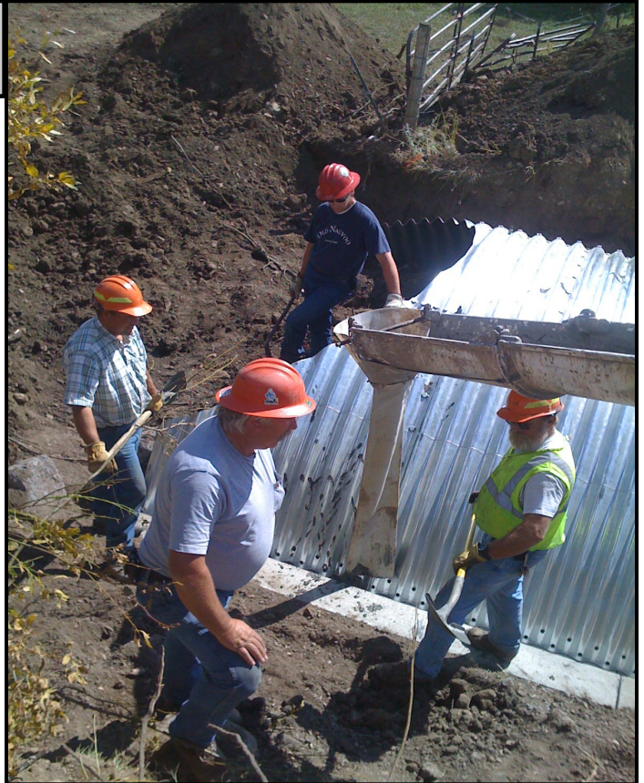
Lee Mabey from the USFS (blue shirt) and crew installing the new culvert on upper Duck Creek. Three other culverts on upper Duck Creek will be replaced in the summer of 2010. Some road closures on Red Rock Road should be anticipated.
