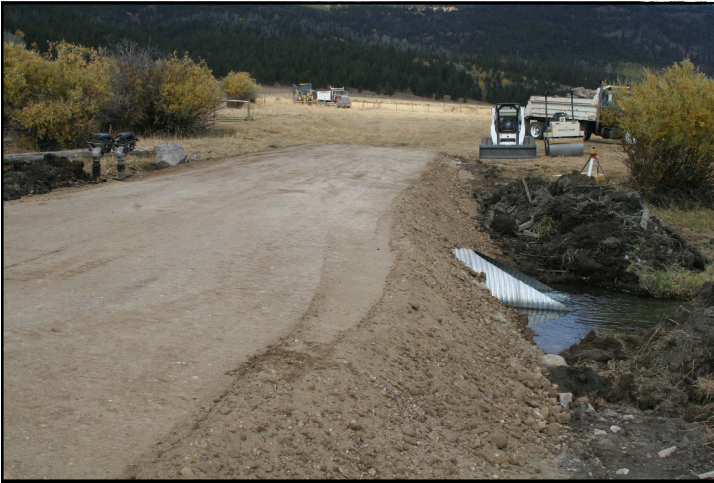
New culvert installation on Spring Creek last summer
