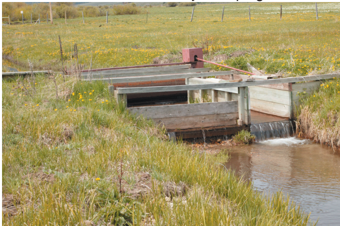
Water diversion with fish screen above on Duck Creek to be updated.
